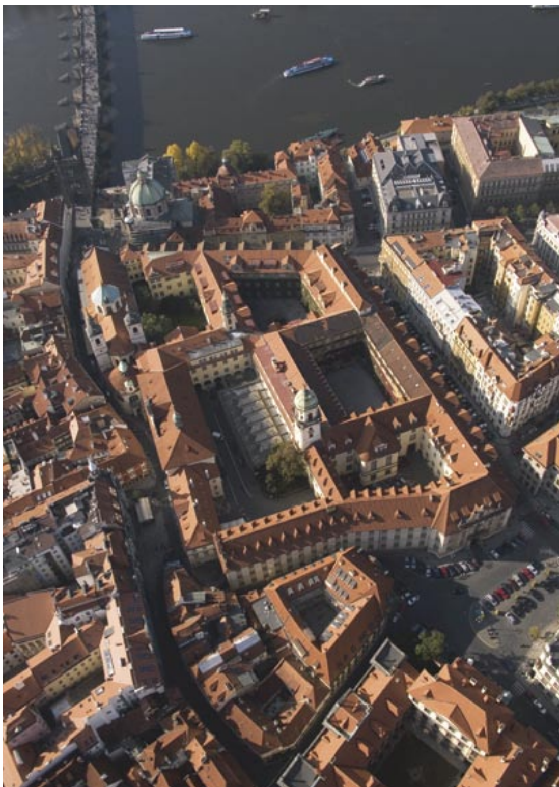
Aerial view of the building of the Klementinum (Photo: Radek Janata)
