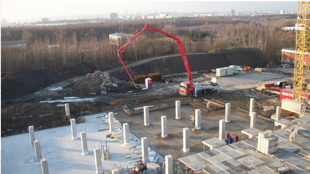
The assembly of prefabricated pillars. Photo: Metrostav, a. s.
