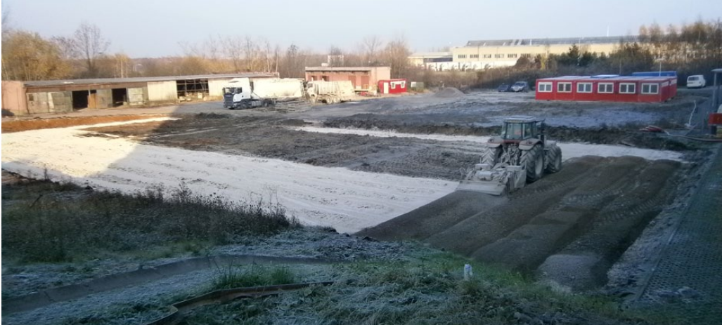
The beginning of the construction work. Photo: Metrostav, a. s.
