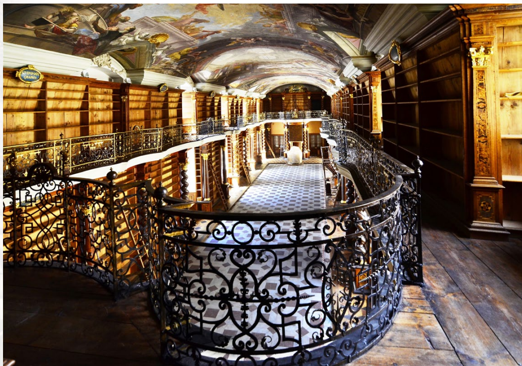
Restoration work in the Baroque Library Hall – restored metal banister. Photo: Pavel Macenauer
